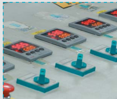
Furnacing process is entirely controlled by the electronic panel which regulates temperature at all steps.
